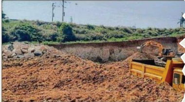
The BDA is preparing groundwork for the railway underpass between Kengeri and Hejjala.
